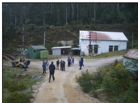
Moorina Power Station.
