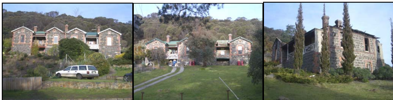
The five cottages built for workmen at the Duck Reach Power Station. The Chief Engineer's house (right) was burnt out in May 2011. Photos: M. Sargent
