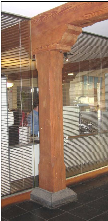
Crown Mills, 22 Cameron St, Launceston: ground, third and fourth levels, showing chamfer-stopped wooden columns reducing in size, cross-heads and beams. Miles Lewis
