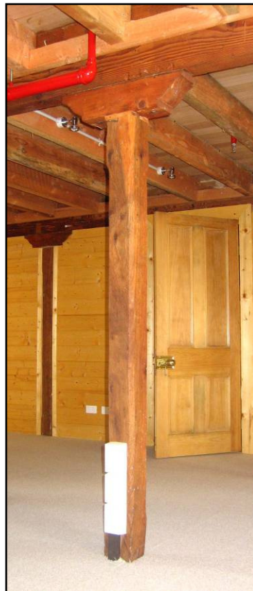
Crown Mills, 22 Cameron St, Launceston: ground, third and fourth levels, showing chamfer-stopped wooden columns reducing in size, cross-heads and beams. Miles Lewis
