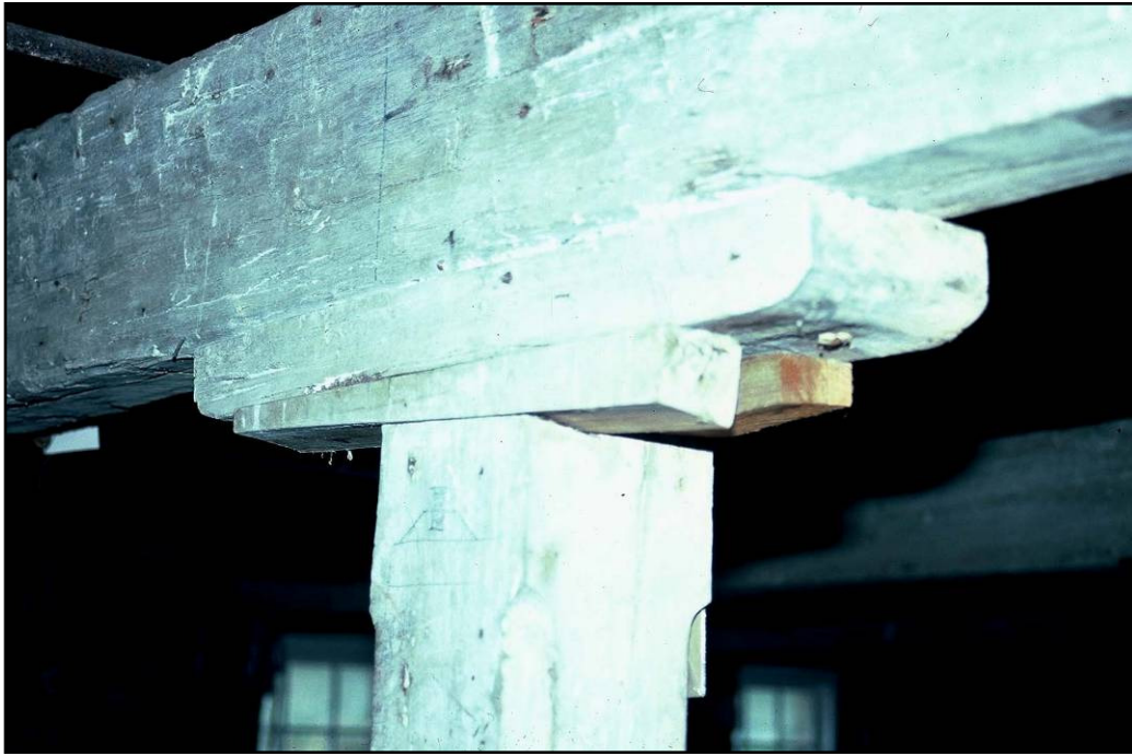
Portarlinton Flour Mill, Turner Court, Portarlinton, Victoria, by Andrew McWilliams, 1857, showing an adzed beam, a cross-head or spreader, modern wedges, and a square chamfer-stopped column. Miles Lewis
