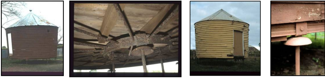
Springall's patent vermin-proof stores in Victoria: Left: 'Ripple Vale', view and substructure. Right: 'Mount Hesse', steddle and view. Miles Lewis.
