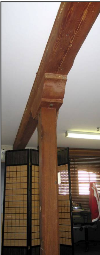
Crown Mills, 22 Cameron St, Launceston: ground, third and fourth levels, showing chamfer-stopped wooden columns reducing in size, cross-heads and beams. Miles Lewis
