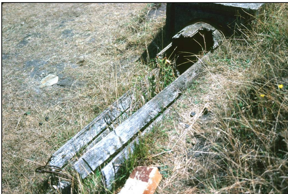
Wood stave pipe, Maria Island Cement Works, Tasmania. Miles Lewis
