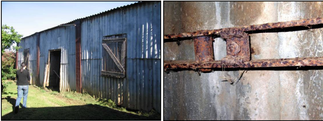
The Edwin Maw building at 'Longford House', Longford: view and girt detail. Miles Lewis
