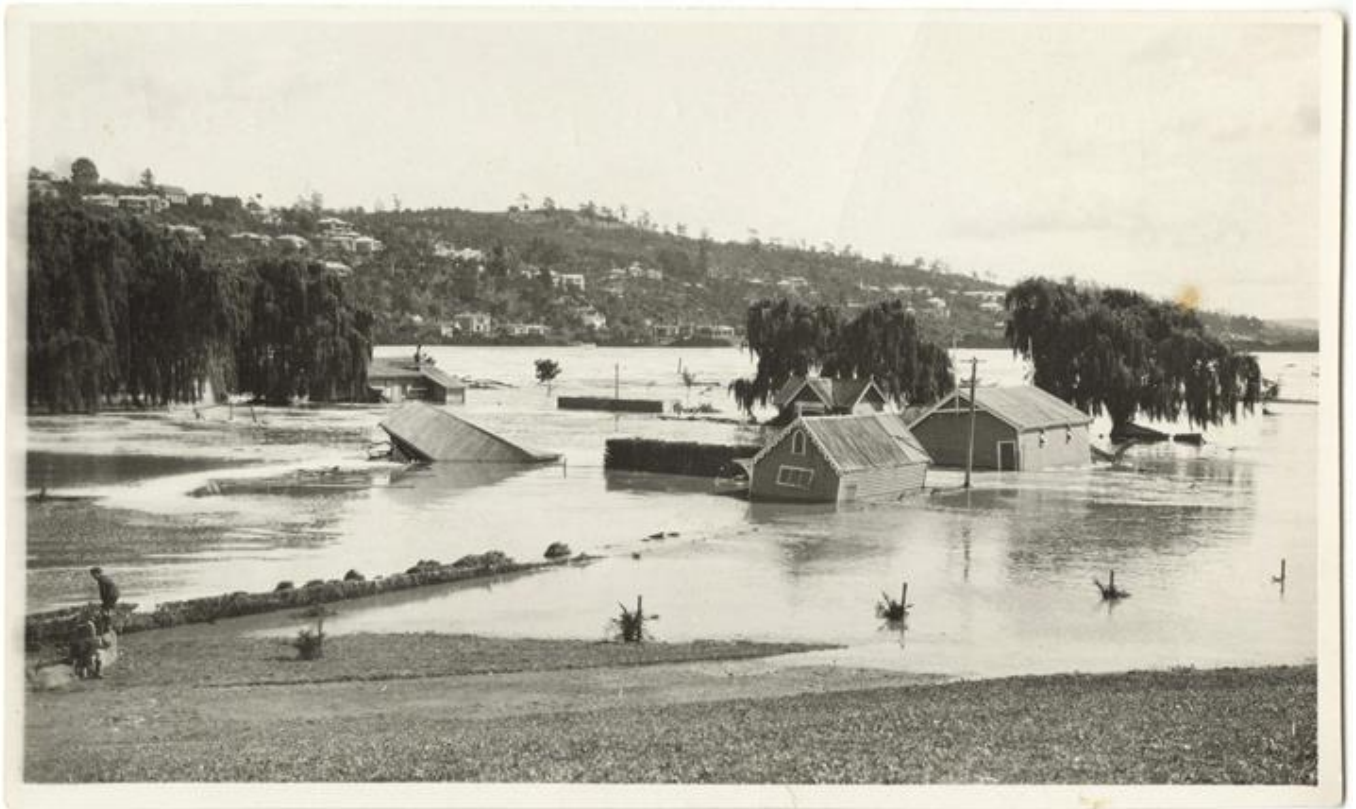
Royal Park during the devastating 1929 floods. Launceston Collection, TAHO, LPIC 84/1/78.
