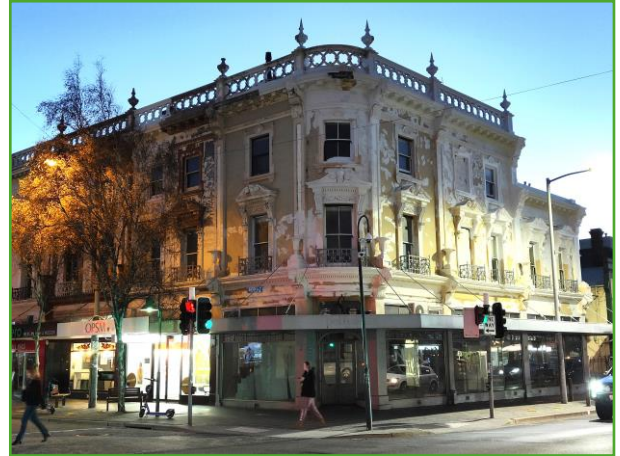
Undergoing extensive renovations in 2024.
